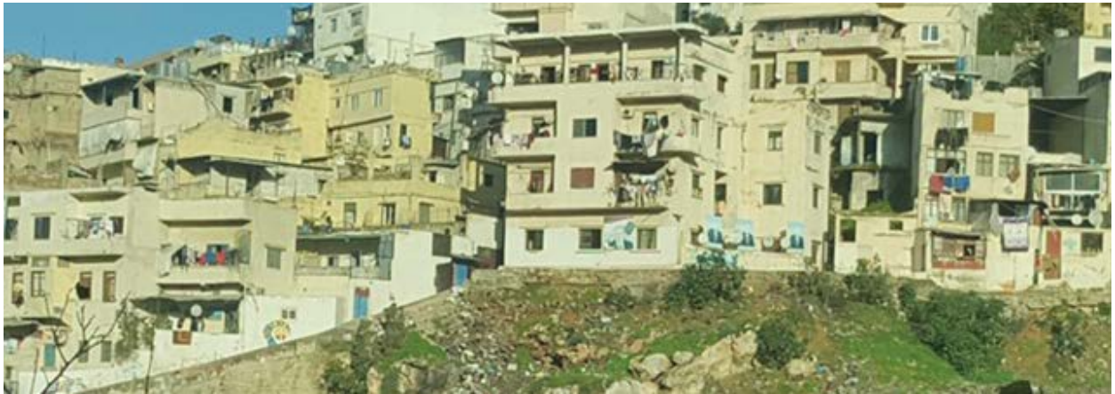
Figure 8-3 Waste Bags Littering Next to Residential Buildings in Remote Areas
